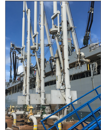
Before Marine Loading Arms replacement at Andersen Air Force Base, Guam.
