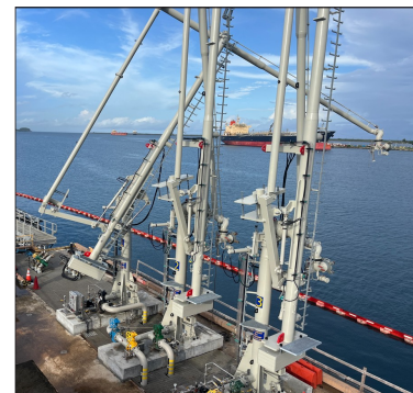
After Marine Loading Arms replacement at Andersen Air Force Base, Guam.
